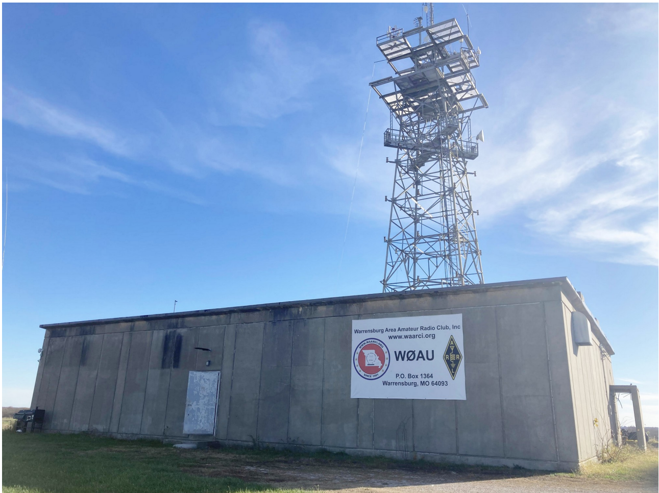
Site base station with 100-foot (minus 50-foot extension) tower, seen from the northwest on the site driveway. The site is owned by the Warrensburg Area Amateur Radio Club, WØAU.
